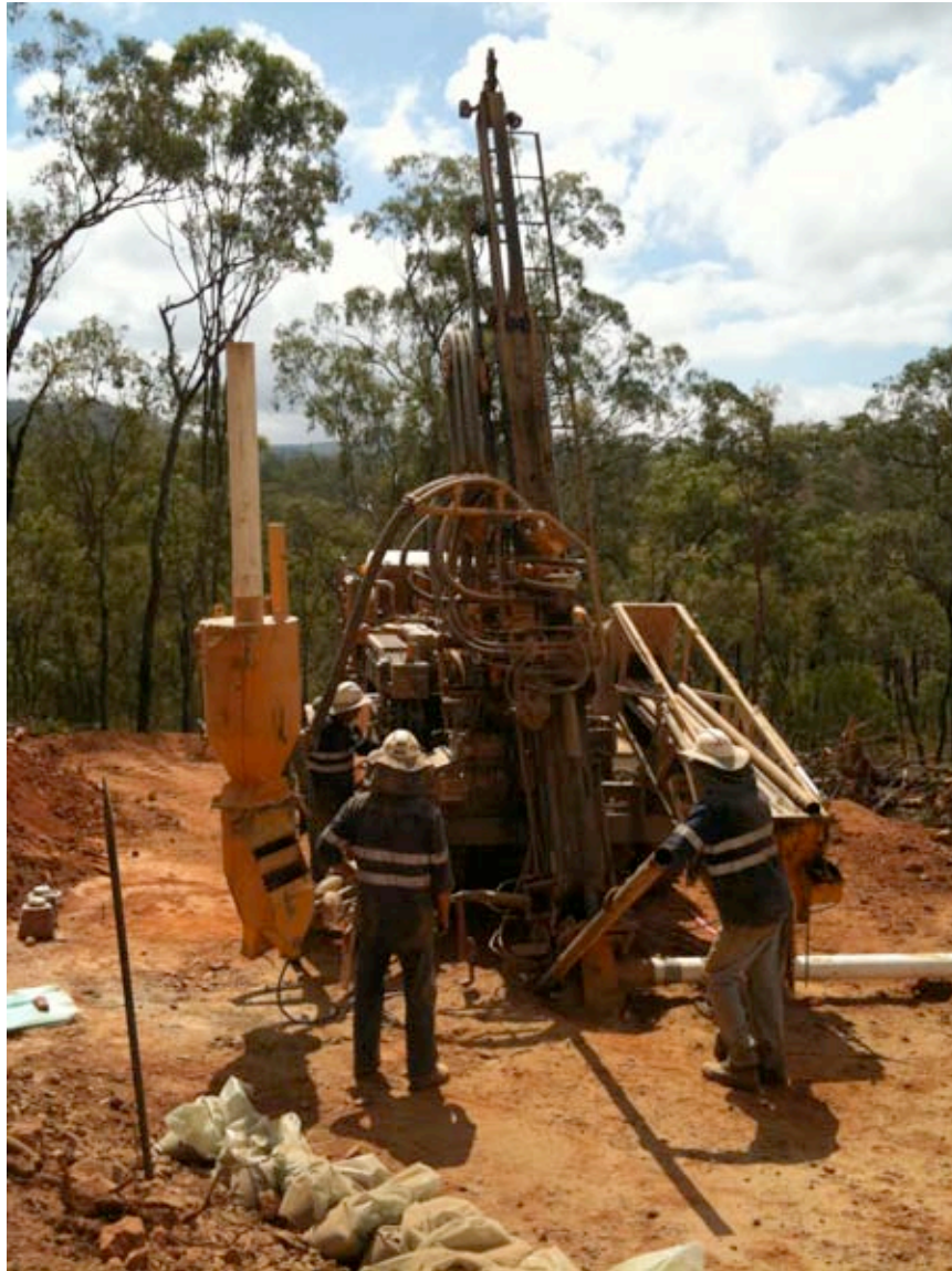
Drilling at Extended September 2011
